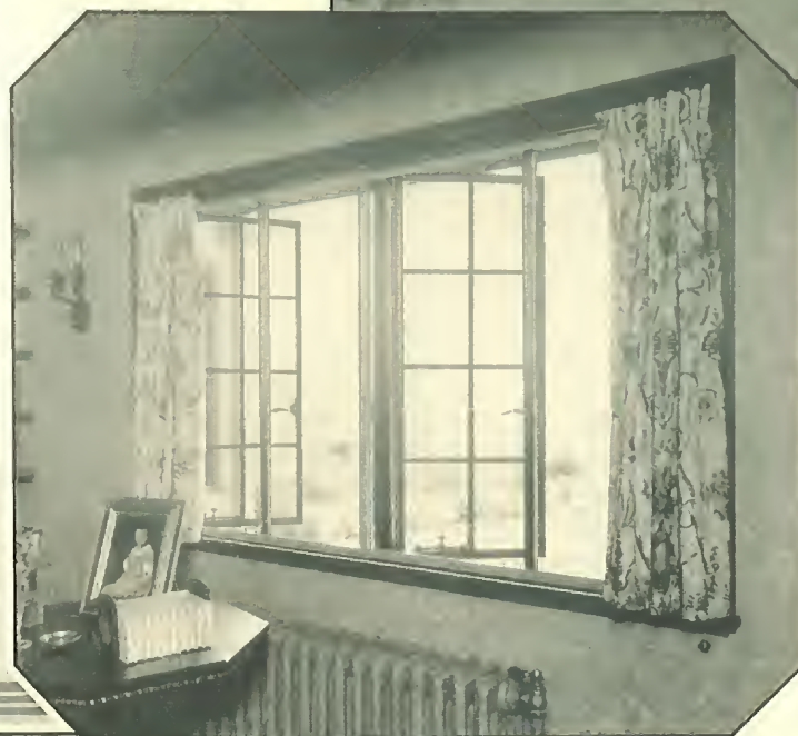
(Right)—There is no interference with drapes and shades in this living room group of casements. Screens sliding horizontally by one another give easy access to window hardware and furnish no barrier to sun or air.
